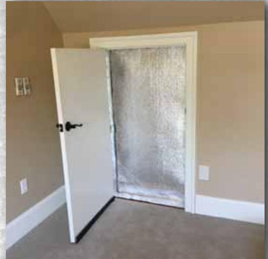
**PRODUCT DIMENSIONS & DESCRIPTIONS:** Double sided scrimmed aluminum foil laminated to polyethylene foam (1/4" nominal thickness)
